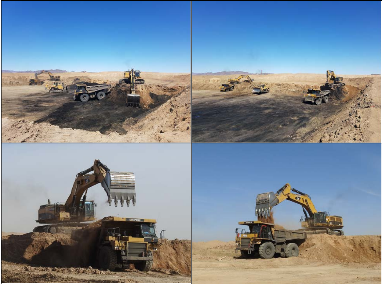
Images: Commencement of BNU Pit 3 boxcut
