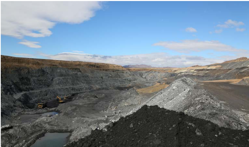
Figure 5 - BNU Pit 1 nearing completion in September 2015
