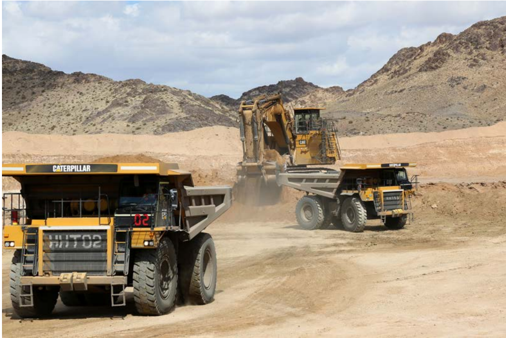
Figure 2 - CAT 6030 Excavator loading CAT 777D trucks stripping overburden from Pit 2
