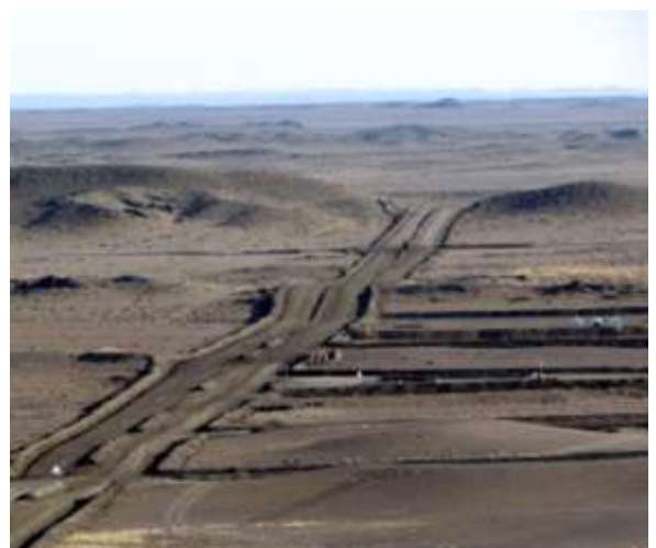
Figure 5: Haul road constructed by Guildford over which ROM coals will be delivered to China for further processing. Source: Guildford
