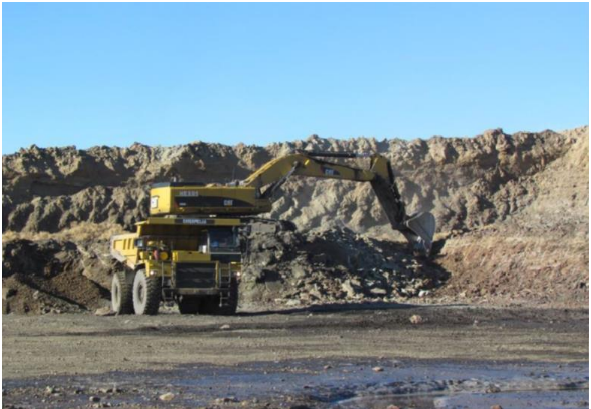
CAT 6030 excavator loading CAT 777D haul trucks on 1604 RL bench
