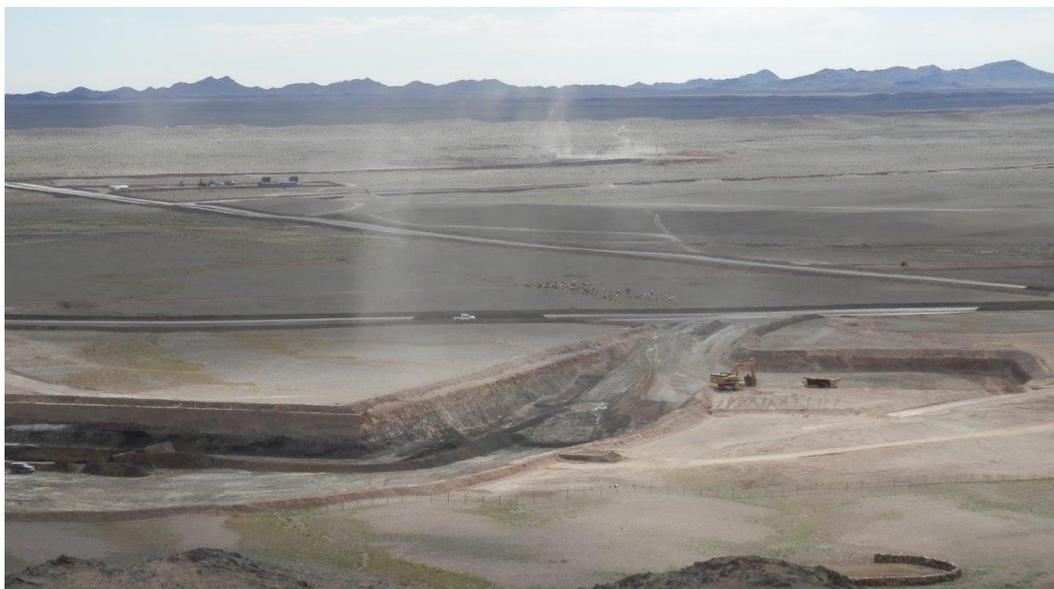
*This photograph shows part of the 3km completed on-lease section of the haul road. Construction will now commence on the 98km off-lease alignment.*
